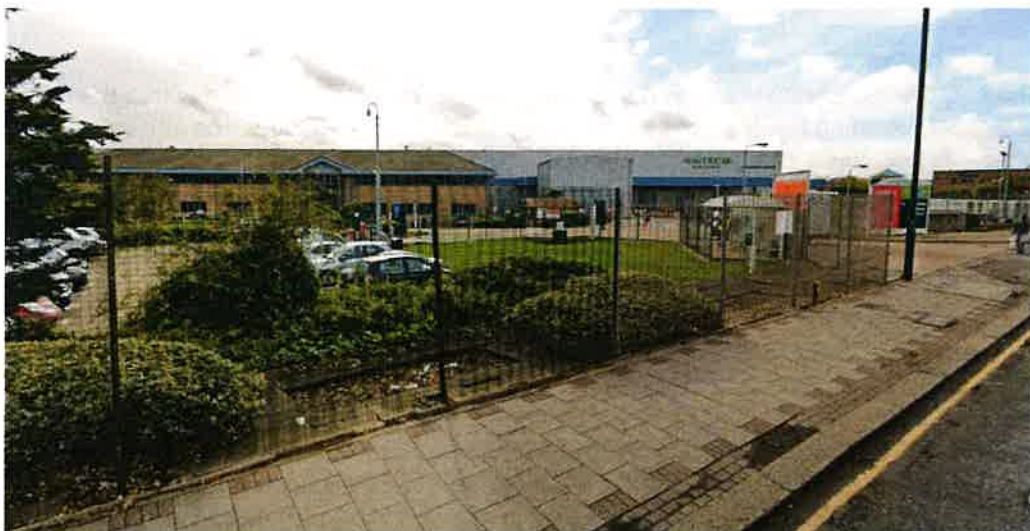
Figure 4: Existing poor streetscape along Southbury Road
